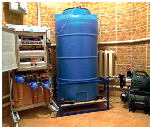
Fig. 6.2.9. EMERALD-UNIVERSAL-500 device as the main universal system for water purification and conditioning in a cottage. When the sensor of the lower level of purified water in the storage tank is triggered, water from the well with a constant flow rate of 500 liters per hour enters the storage tank, having previously passed all the stages of purification in the EMERALD-UNIVERSAL-500 device. When the upper level in the storage tank is reached, the EMERALD-UNIVERSAL device turns off. A pressure boosting station connected to a storage tank and connected to an in-house water distribution system provides the entire cottage with clean water at any time and in any required amount.
